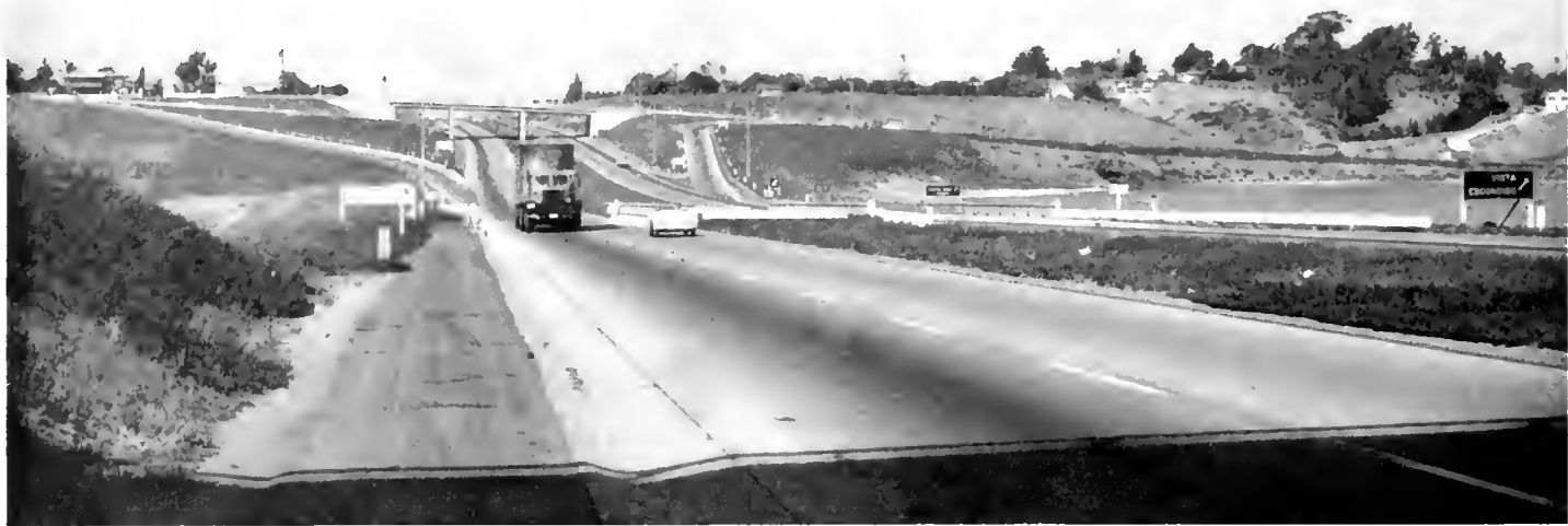
Vista Way separation of junction of US 101 and Sign Route 78 between Oceanside and Carlsbad, showing diamond type ramps
